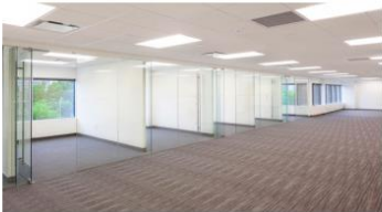
Butt-Glazed Wall with Aluminum Top/Bottom Channel
